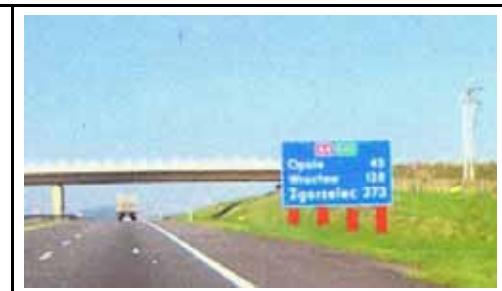
III. Safety supports
