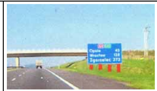
III. Safety supports
