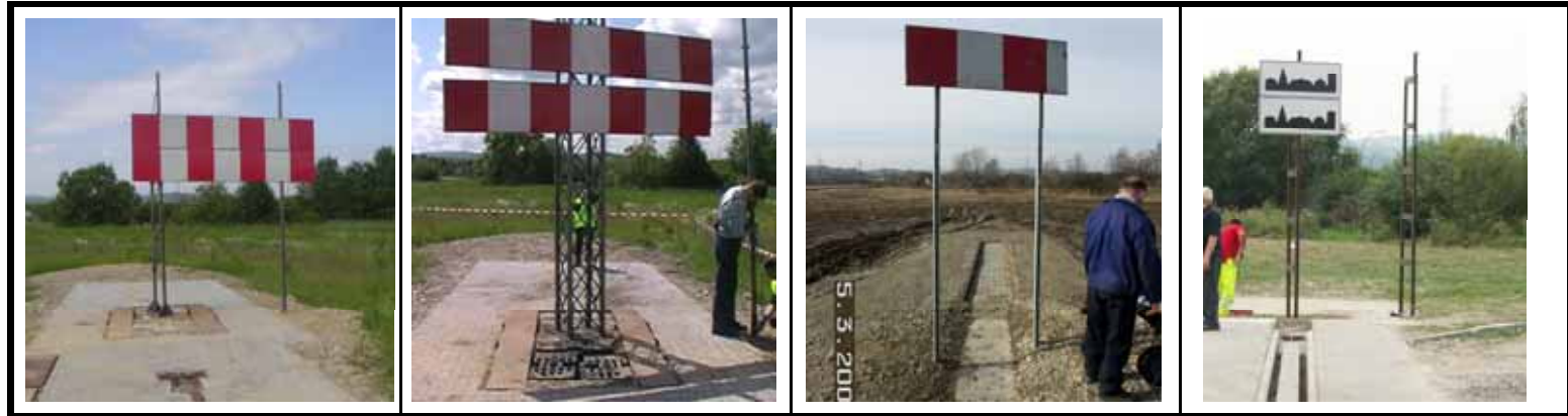
Different sorts of supports on X-307 profile base
